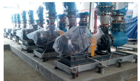
SINGLE STAGE PUMP DETAIL
