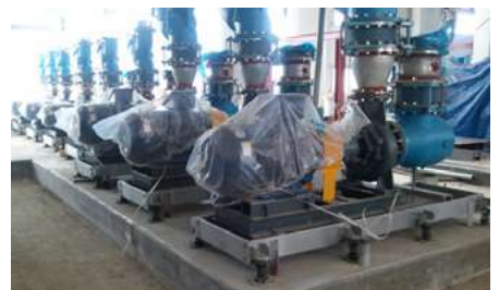
SINGLE STAGE PUMP DETAIL
