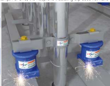
Anti-Vibration Lower Part Welding
