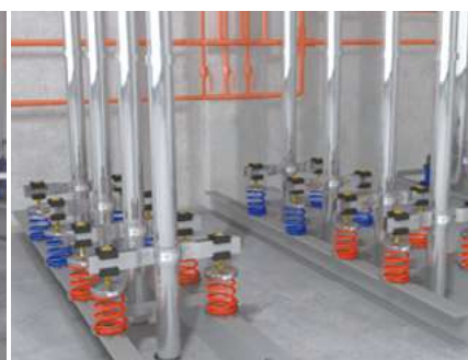
Completion of Anti-Vibration Spring Installation
