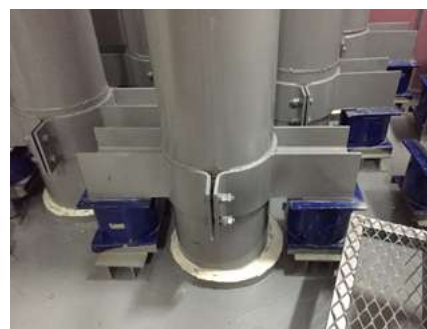
Example of Anchor Bracket Installation
