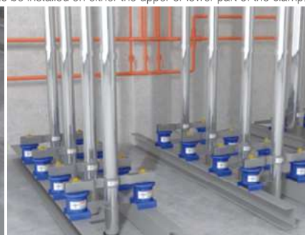
Completion of Anti-Vibration Guide Installation
