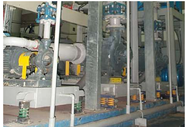
IN-LINE PUMP DETAIL
