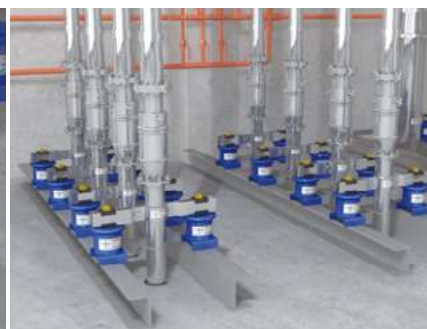
Completion of Anti-Vibration Installation
